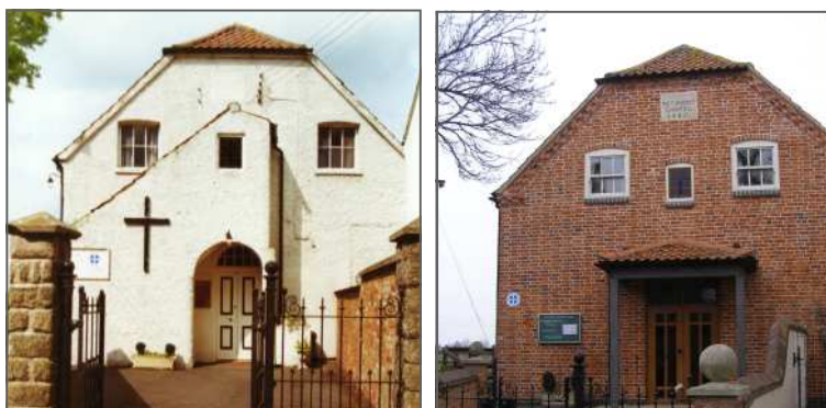
Bottesford PM Methodist chapel before refurbishment - and after! JSI
