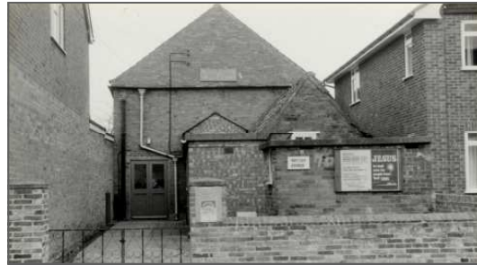
The chapel in use as the school dining room. DCA
